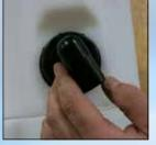
Step 6 Apply thread sealant to 90° barb and hand tighten into top tank bulkhead fitting. Torque 1/2 to 1 full turn with wrench until facing five o'clock position.
