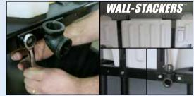
**Step 4** Bolt elbow to the stand's centermost pre-drilled holes.
