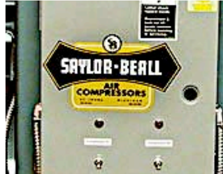
Left: Outside enclosure with toggle switches and run lights.
